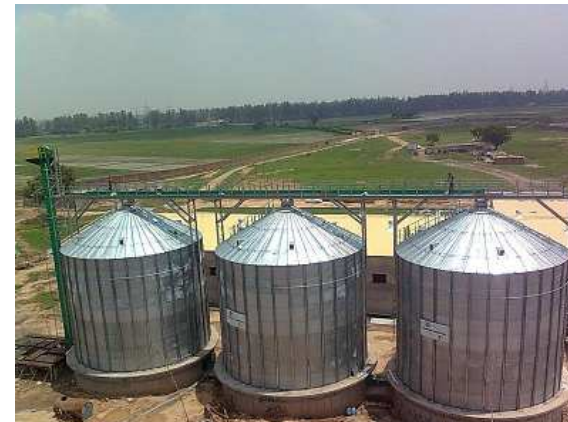
Grain Storage Silo System
